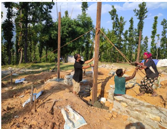
Metal Column Erection
