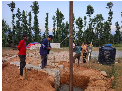
Metal Column Erection
