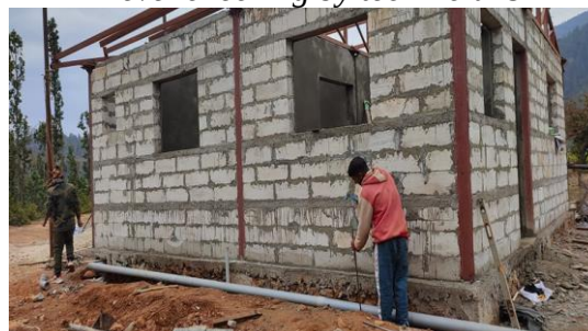
Waste water pipeline works
