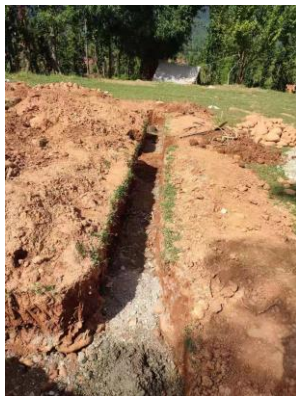
Trench for the Substructure Wall
