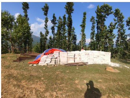
Construction materials at site
