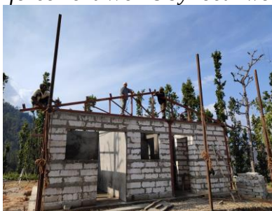
Metal Truss Erection
