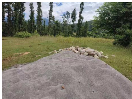
Construction materials at site
