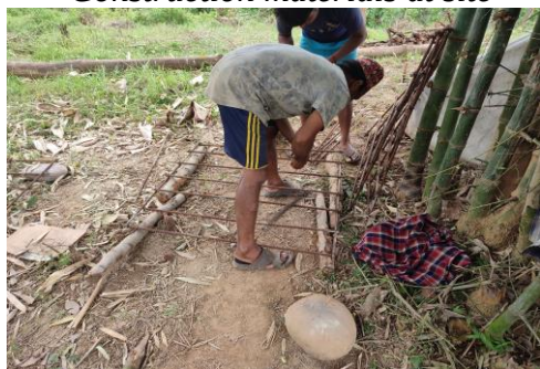
Reinforcement Works by local workers
