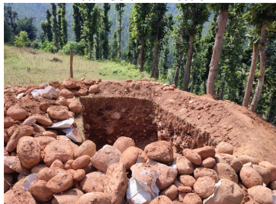
Excavation works for the Septic Tank
