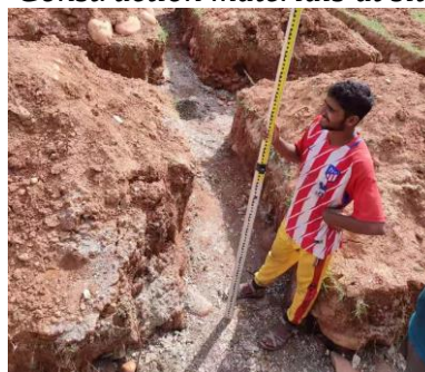
Level checking by technicians
